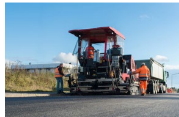
| Asphalt Binder Analysis
